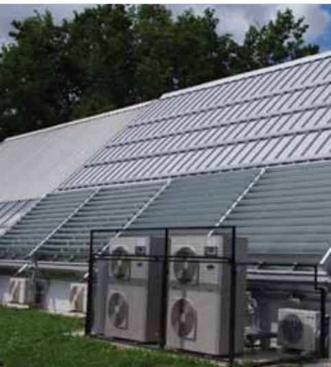
karantenski rastlinjak s podtlakom quarantine greenhouse with negative pressure
